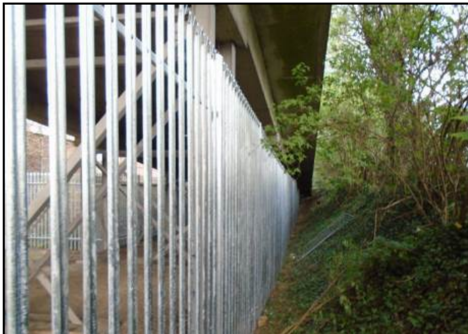
Figure 3 - fence tapering to lowest level under ramp
